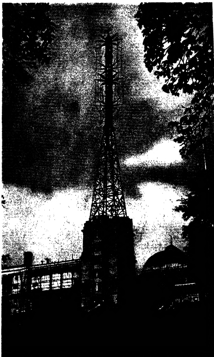
Frontispiece: THE AERIAL TOWER OF THE B.B.C. TELEVISION TRANSMITTER AT ALEXANDRA PALACE, NORTH LONDON (Courtesy of the B.B.C.)
