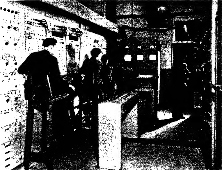
FIG. 1.10B. CONTROL ROOM "A" OF THE B.B.C. TELEVISION STATION
