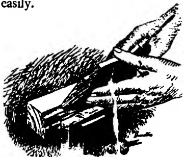
Fig. 23. Small moulding plane in use.
