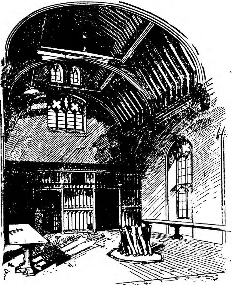
Fig. 3. This magnificent example of the mediæval craftsman's art embodies principles which are still used in modern joinery. The illustration shows the beautifully constructed 14th century timber roof of Penshurst Place, Kent. (Reproduced by courtesy of C. H. Hayward.)
