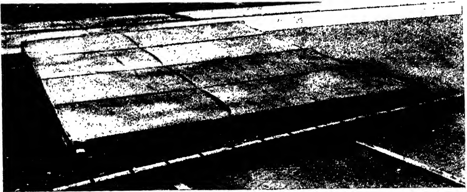
FIG. 99(a).—WOOD CURING FRAME COVERED WITH TARPAULIN OR WATERPROOF PAPER.
