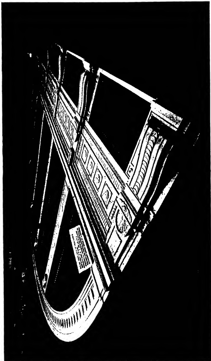
PLATE 20.—This large casting, 60 ft. wide by 43 ft. high, consists of a window surround, mullions and panels for the Plaza Constitución Station, Great Southern Railway, Buenos Ayres.
