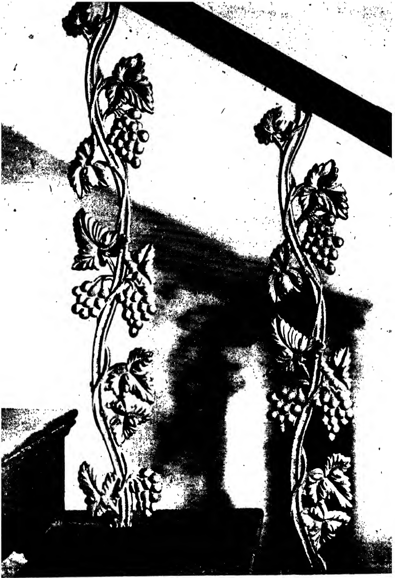
PLATE 23.—Decorative cast iron balusters at the De Grey Rooms, York. (Reproduced by courtesy of the National Buildings Record.)
