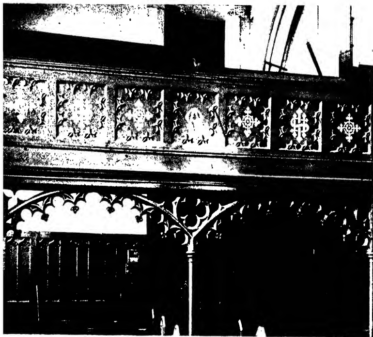
PLATE 22.—Cast iron arches supporting the gallery front of St. George's Church, Birmingham. (Reproduced by courtesy of the National Buildings Record.)
