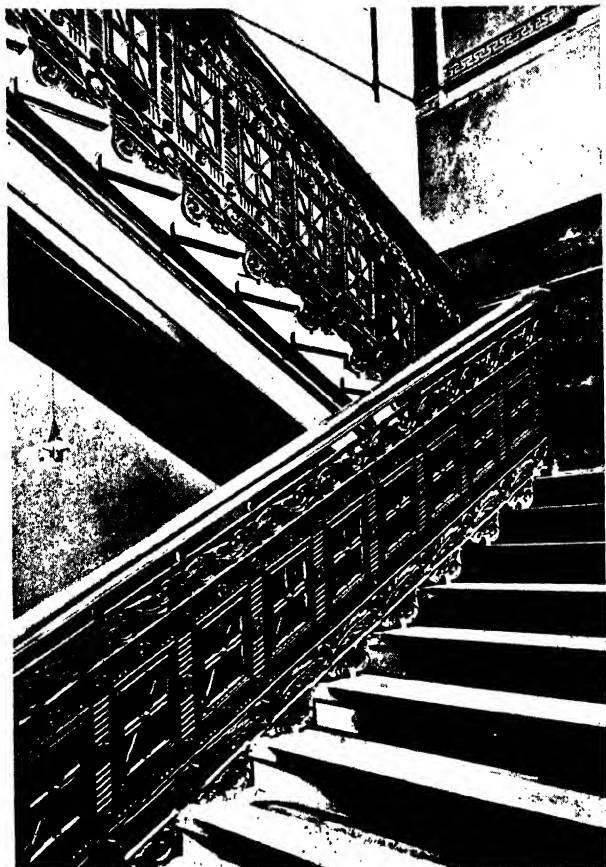
PLATE 24.—Cast iron balustrade on the staircase of St. Andrew's Halls, Glasgow.
