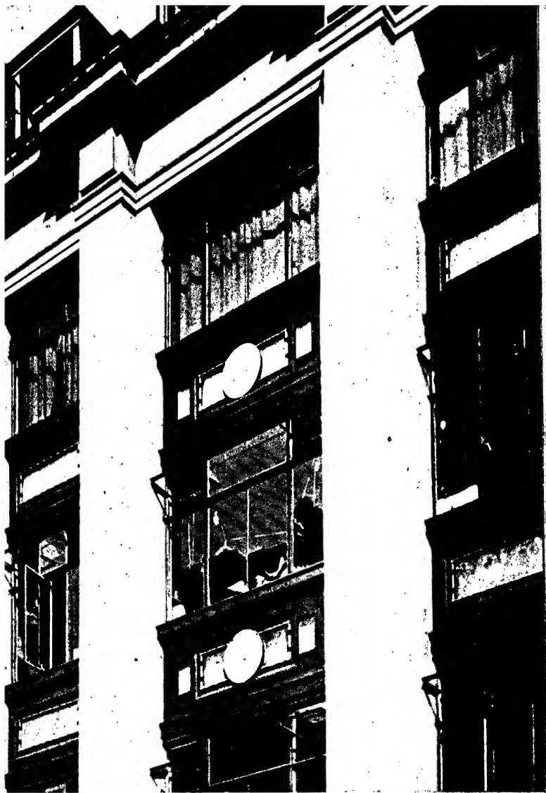
PLATE 17.—Cast iron window breast panels on the façade of a building in d'Arblay Street, London, W.C.1. Architects: Abbot and Dickens.
