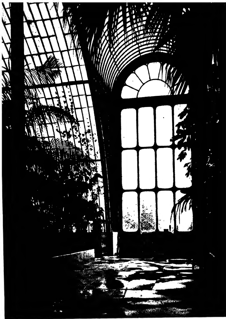
PLATE II.—The interior of the Palm House at Kew Gardens, designed by Decimus Burton and Richard Turner. Begun in 1844, this structure was an example of the use of cast iron and glass units. (Reproduced by courtesy of the Architectural Press , from Glass in Architecture and Decoration , by Raymond McGrath and A. C. Frost.)
