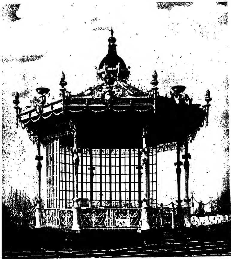
PLATE 35.—A typical example of the highly ornamental use of cast iron in the late nineteenth century. A bandstand at Southend-on-Sea.
