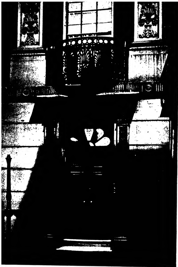
ATE 28.—Cast iron balcony on a house in the Adelphi, London, designed by Robert Adam. (Reproduced by courtesy of F. R. Yerbury.)
