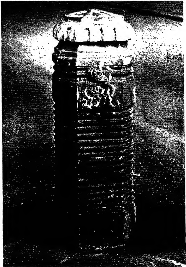
PLATE 30.—Cast iron bollard in Hyde Park, London. Here is an example of the decorative treatment of a casting giving additional structural strength, as well as lightening the general appearance.
