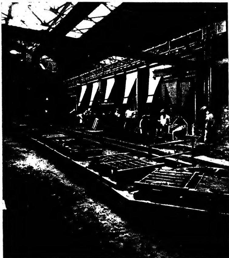
PLATE I.—Mechanization in a modern foundry. This shows the sand plant, push-plate conveyor, sand hoppers, casting runway and mould conveyor.
