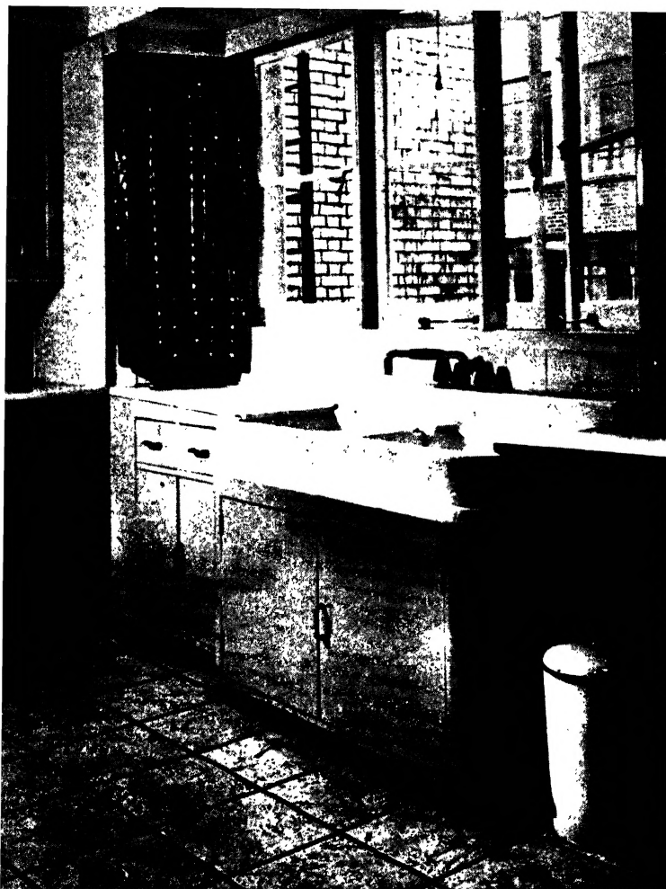
PLATE 48.—A kitchen installation, with a sink, draining-board and splash-back tiles of cast iron.
