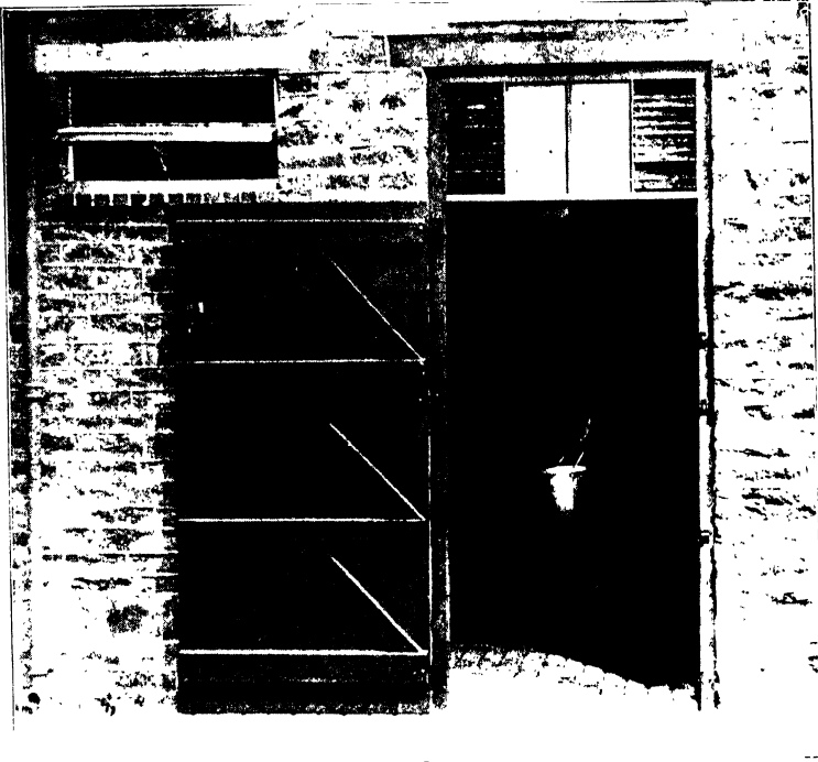
Fig. 27. Water bucket fixed to door of box.
