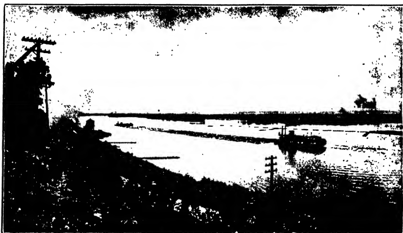
FIG. 259.—The Mississippi—a wasted waterway. It will probably be used much more than it now is as freight costs rise and we develop a national organized system of transportation. Looking south from Alma, Wisconsin. Railroad tracks, water tank, Mississippi stern wheeler, log raft, tug. Wing dams—a device much used in Europe to narrow the current, deepen the water and also make the water dig the channel deeper. (Courtesy H. Burgess, Corps of Engineers, U. S. Army.) (From North America , published by Harcourt, Brace and Company.)
