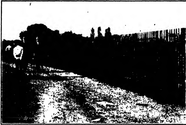
FIG. 185.—German fence made of forest thinnings. Uprights are first thinning 1\frac{1}{2} – 2\frac{1}{2} inches in diameter, round. Cross pieces are second thinning, split. Posts are larger round pieces. No sawdust or slab waste. The forest was planted with trees about as far apart as hills of corn in American fields. (Photo, J. Russell Smith.)
