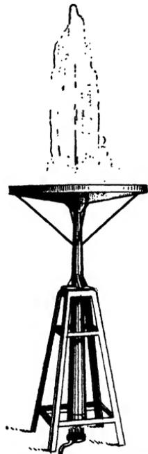
FIG. 203.—Apparatus for simulating geyser action in the lecture room (by courtesy of Professor B. W. Snow).
