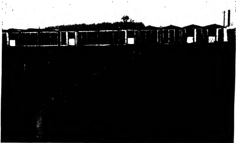
FIG. 22. Double-light span range prepared for receiving the lights. Note the low earth ridge
