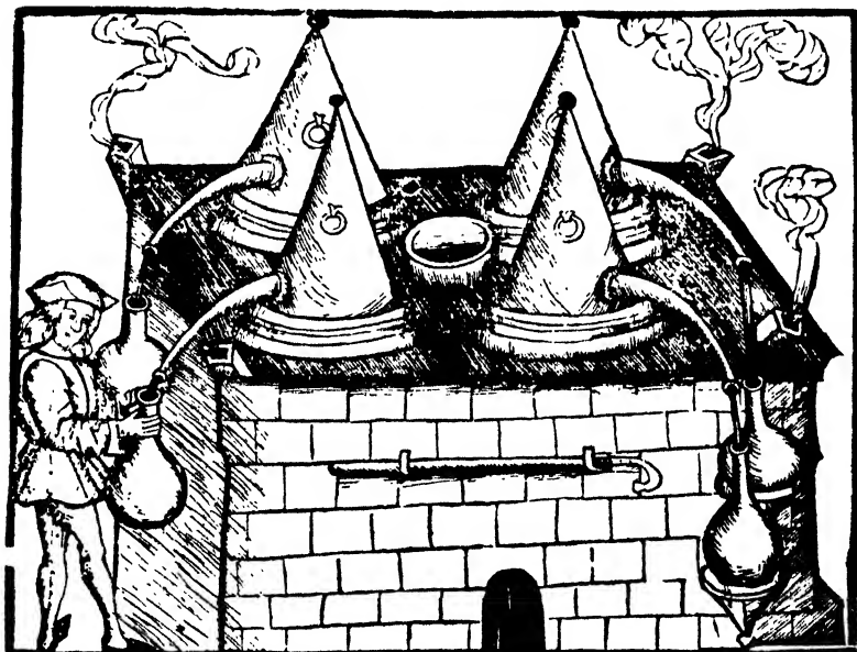
9. 'Ane boy that kept the furnes fire.' A furnace and stills with Rosenhut condensers. From Das Buch zu Distillieren , H. Brunswick, Strassburg, 1519
