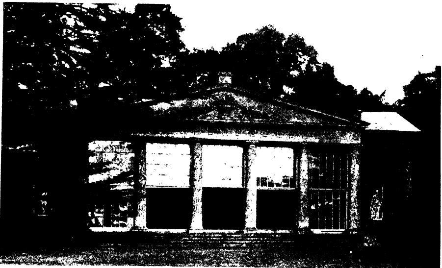
83 Croome Court, Worcestershire: the Doric Orangery (after 1760)
