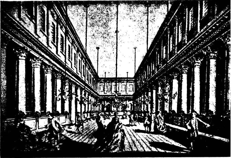
23 Assembly Rooms, York. Built by Lord Burlington (1730-2) in the strictly Palladian style
