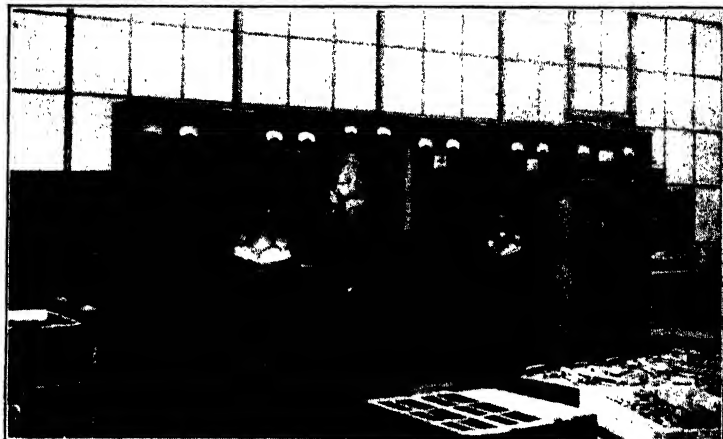
Typical large Hewittic rectifier for mass charging of batteries.
