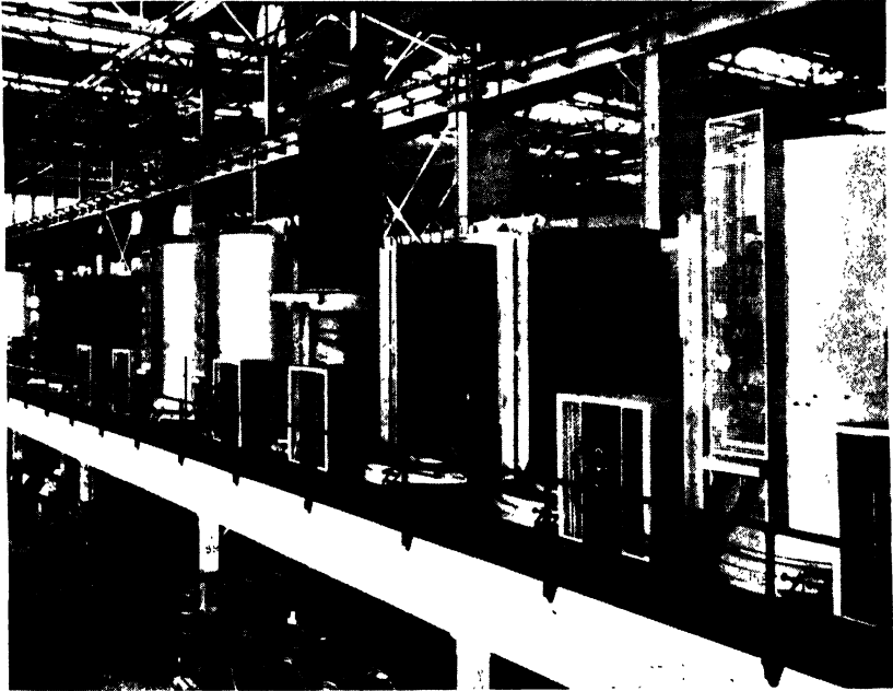
FIG. 78. Battery of bell-type furnaces of the design shown in Fig. 77, installed at the plant of the Ford Motor Company. Each bell takes two coils of 52-in.-wide sheet. Each coil weighs 16,000 lb. The furnace battery consists of 37 bells and 111 bases. (Courtesy Westinghouse Elec. Corp.)
