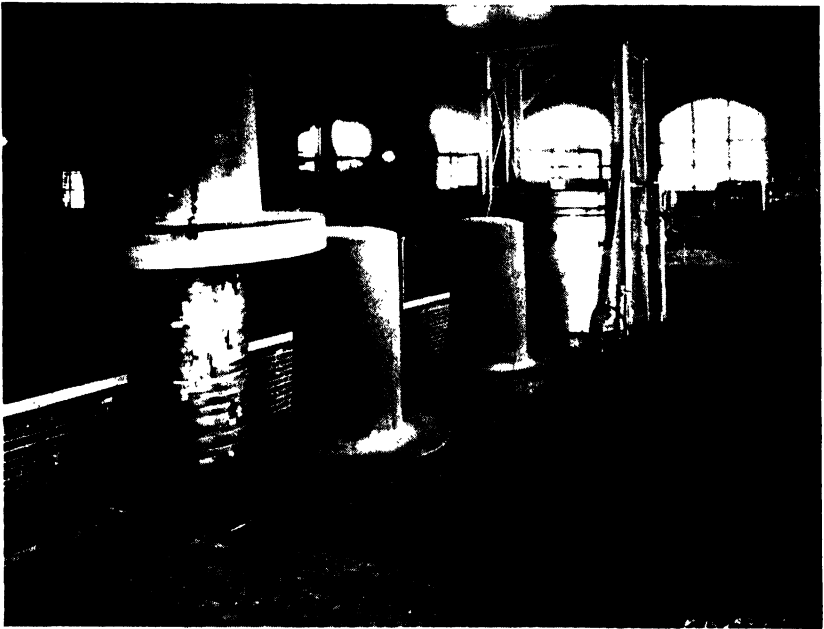
FIG. 92. Bell annealing of coiled strip. (Courtesy Westinghouse Elec. Corp.)
