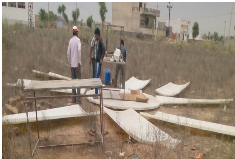
Figure 6. 6 Assembling GRP panels
