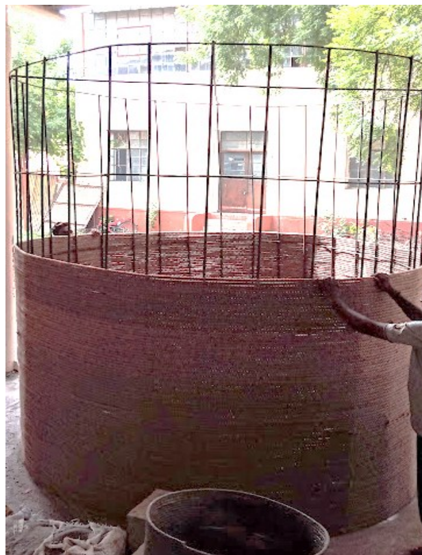
Figure 4. 6 Winding jute fibre to the frame
