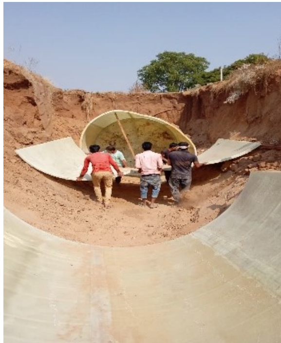
Figure 6. 9 Assembling GRP panels of directional tunnel
