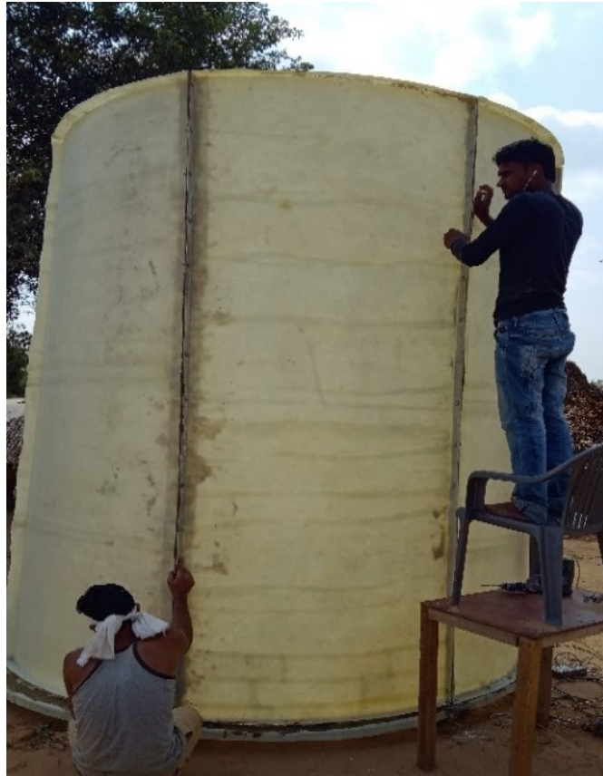
Figure 4. 12 Assembling multiple panels for GRP water tanks
