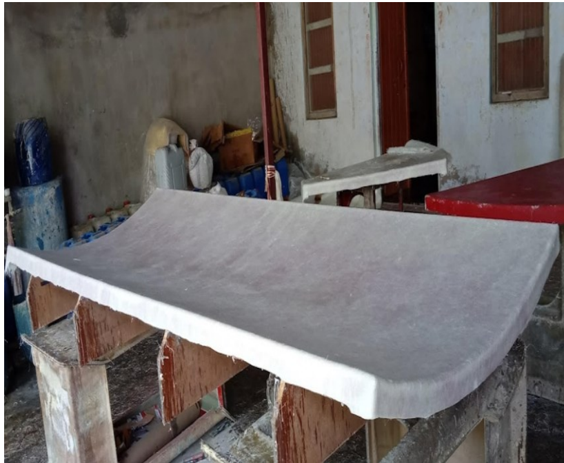
Figure 4. 10 GRP panels set for curing
