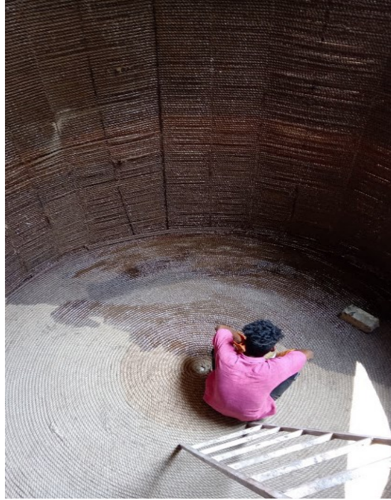
Figure 4. 7 Internal application of epoxy resin-hardener mixture coat
