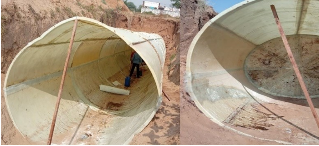
Figure 6. 10 Strengthening of directional tunnel at analysed failure points during execution
