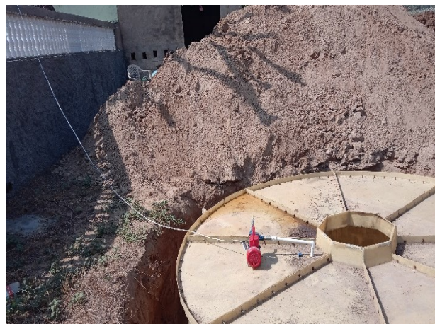
Figure 6. 12 Installation of solar water pump at a household GRP water tank
