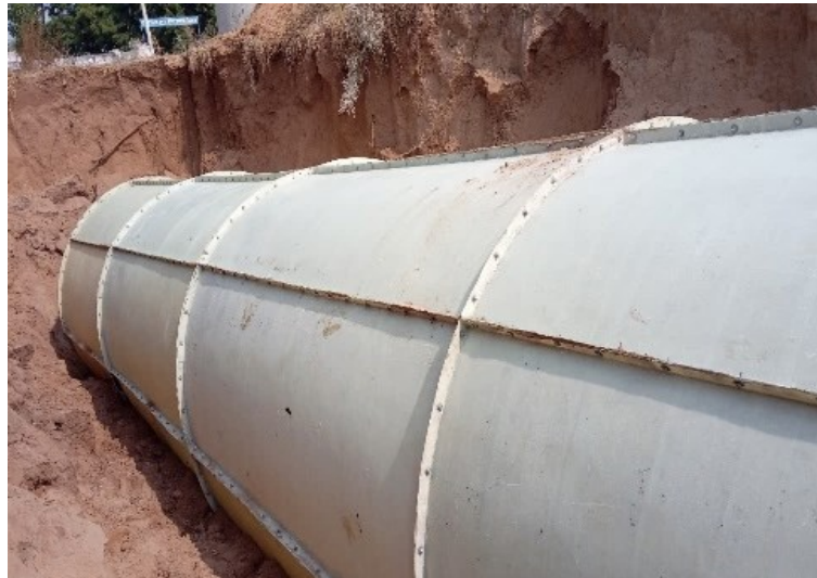
Figure 6. 11 Final directional tunnel
