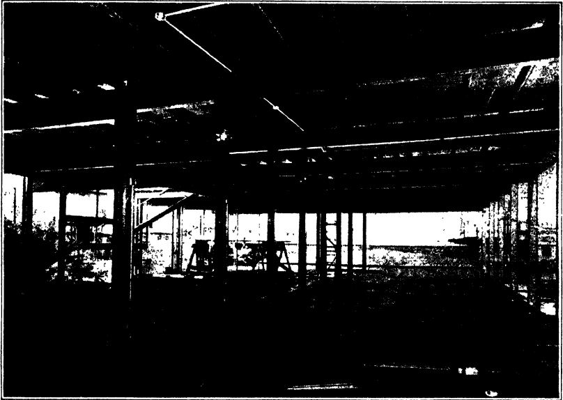
Fig. 177. Battledeck Floor in an Office Building Courtesy of Lincoln Electric Company, Cleveland, Ohio
