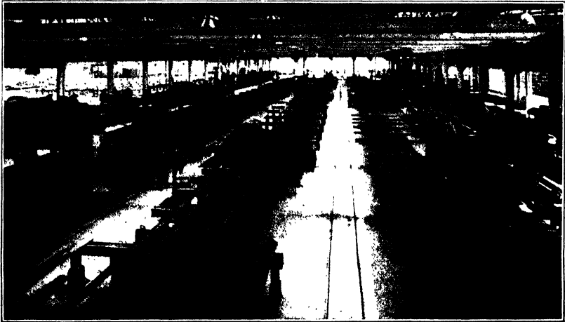
Fig. 41. New Structural Steel Fabricating Shop, Moore Drydock Co., Oakland, California Courtesy of Thomas Machine Manufacturing Company, Pittsburgh, Pennsylvania
