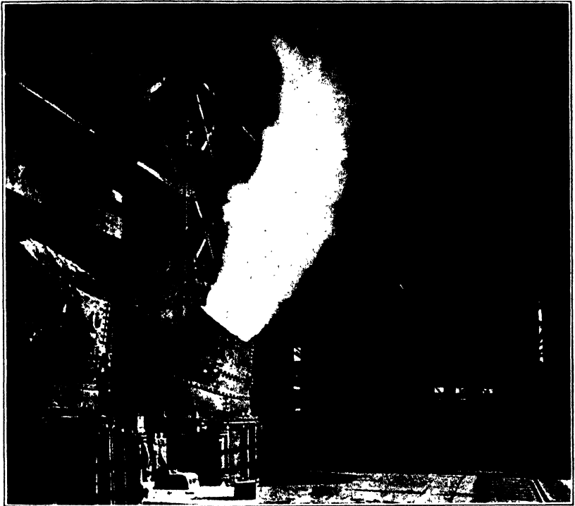
Fig. 7. Bessemer Converter in Operation Photo by Bethlehem Steel Company
