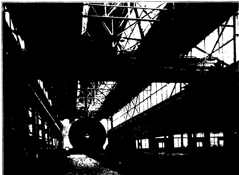
Fig. 155. Crane Girder Runways Supported on Independent Columns Courtesy of Whiting Corporation, Harvey, Illinois
