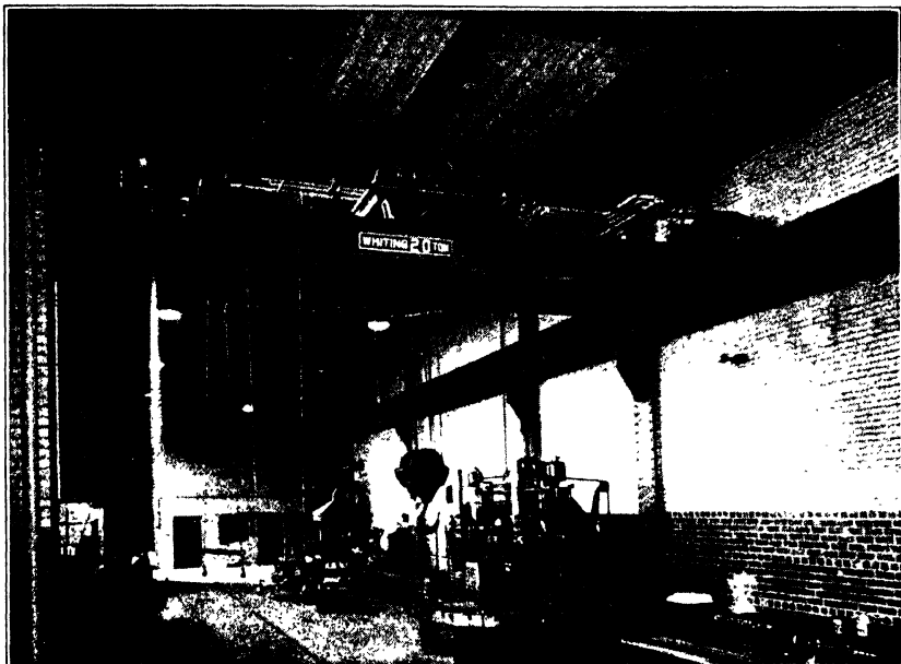
Fig. 154. Crane Girder Runways Supported on Brackets Courtesy of Whiting Corporation, Harvey, Illinois
