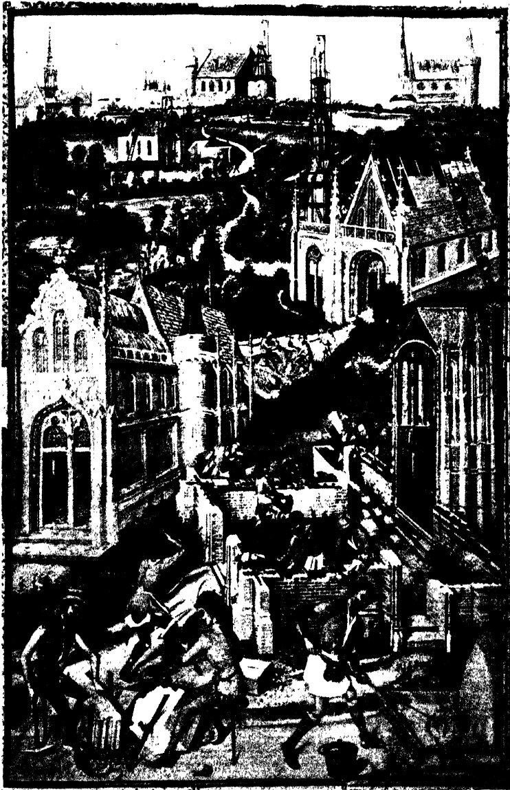
16 FIFTEENTH-CENTURY BUILDERS AT WORK. Notice in the Foreground the Mortar-Mixer, the Bricklayers, and the Masons cutting Moldings on Stone Blocks
