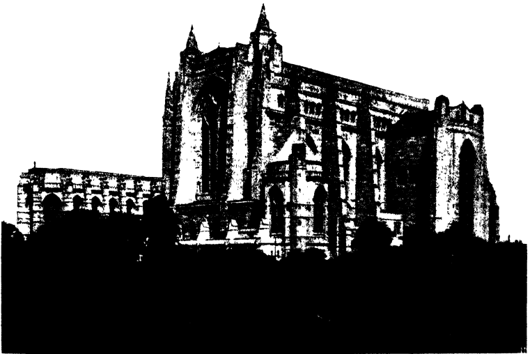
132 LIVERPOOL: The Completed Quire and Lady Chapel of the New Cathedral. Sir Giles Gilbert Scott, R.A., Architect
