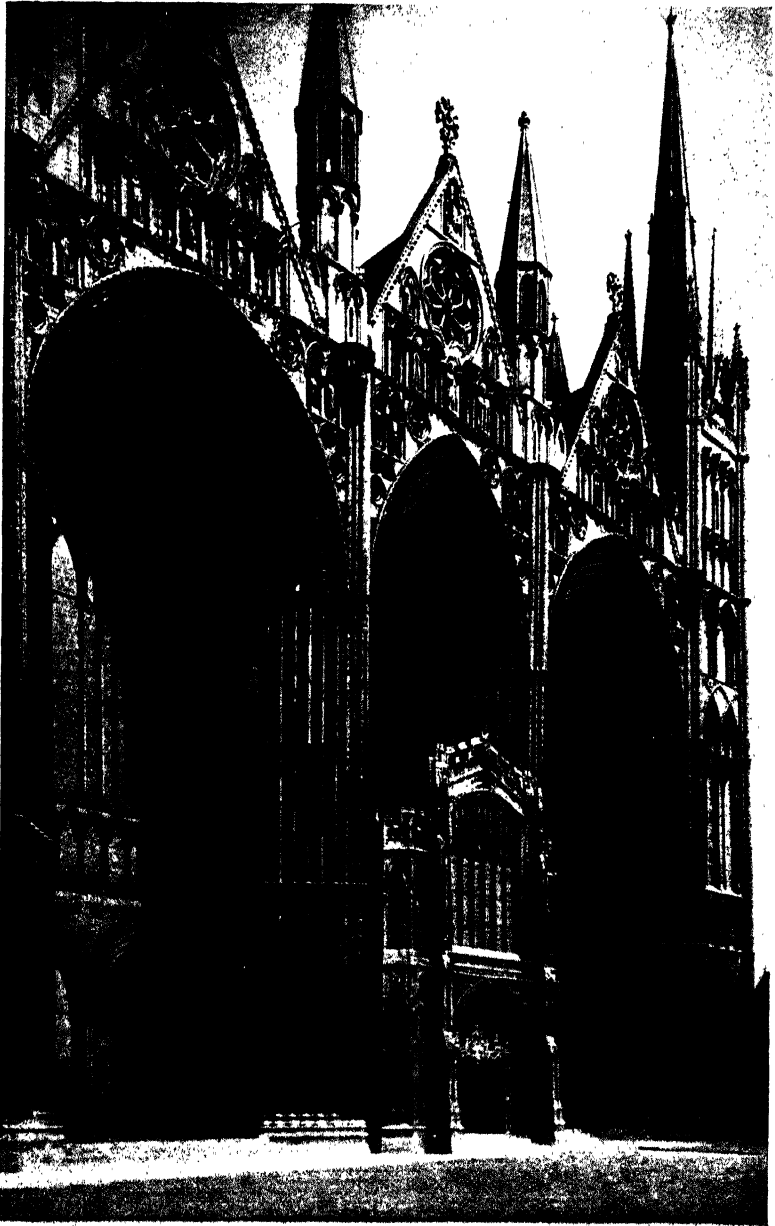
79 PETERBOROUGH: The Great Arches of the West Front. The little Porch in the centre is a Fifteenth-Century Addition
