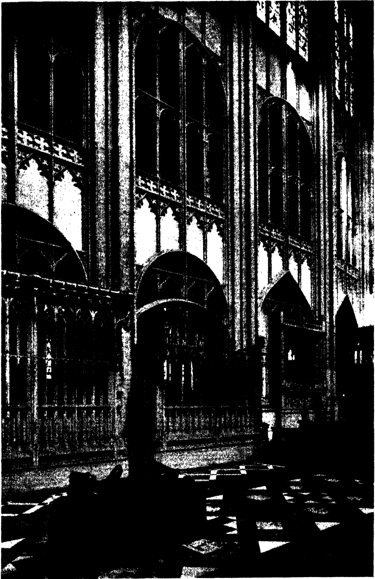
8 GLOUCESTER: A Detail of the Quire Reconstruction that worked the Perpendicular Revolution. The old Norman core is overlaid with a delicate rectilinear scaffolding of light masonry. The shrine of Edward II can be seen screened off in the central bay, and in the foreground is the early effigy of Robert of Normandy
