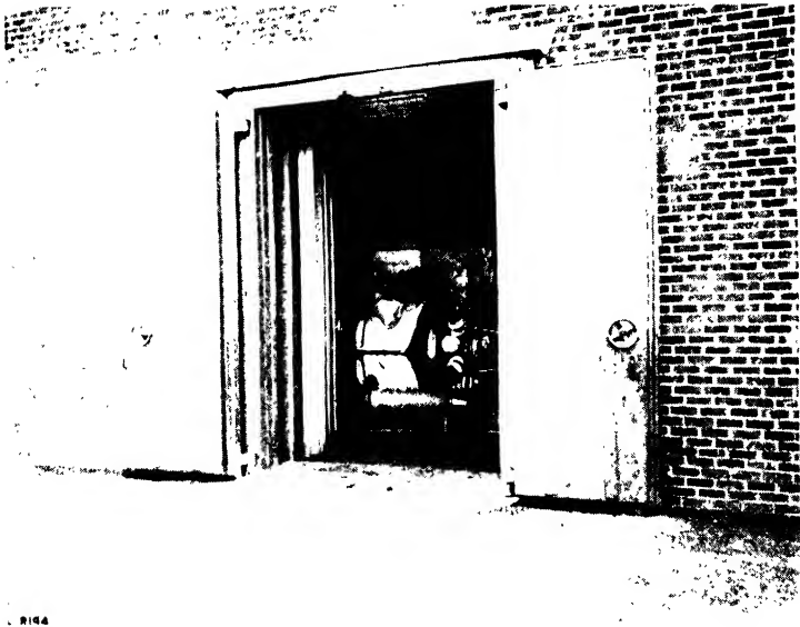
FIG. 331 - The side entrance to the engine room with its double sound-proofed doors
