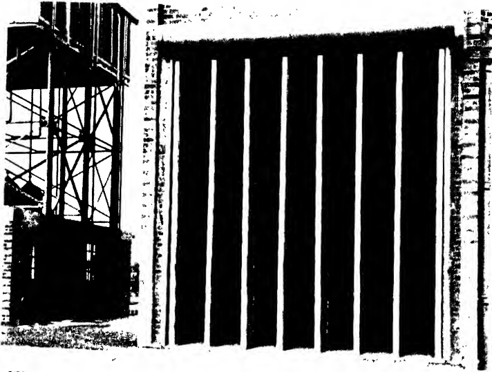
FIG. 332 Exit of exhaust tunnel, showing the specially shaped sound absorbing panels.
