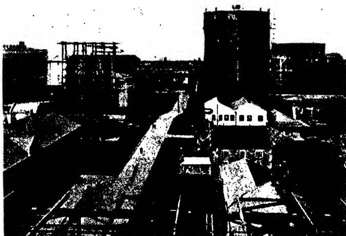
FIG. 48.—Part of Synthetic Ammonia Works at Billingham.
