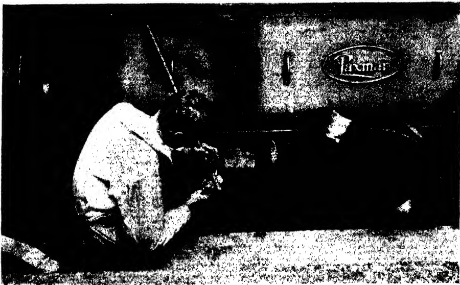
Fig. 1K. —PREPARATION FOR FINAL BOLTING DOWN Note attachment of depth irons.
