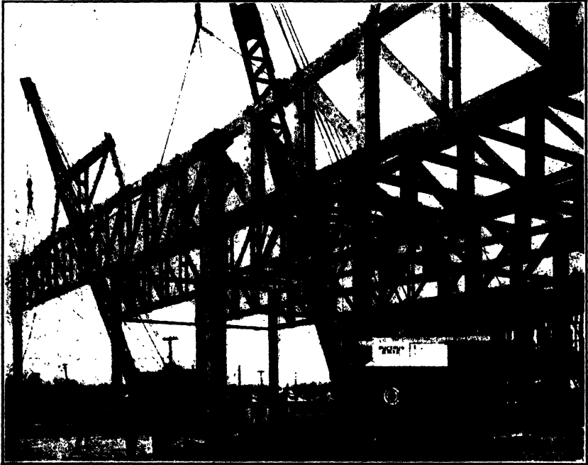
FIG. 159. Typical Timber Truss Construction.
