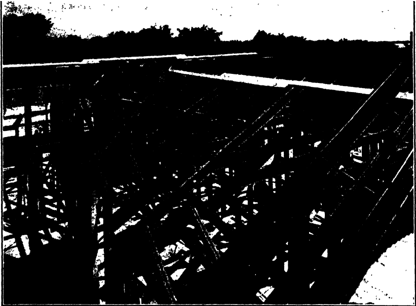
Fig. 189. Typical Roof Framing with Stran-Steel Sections.
