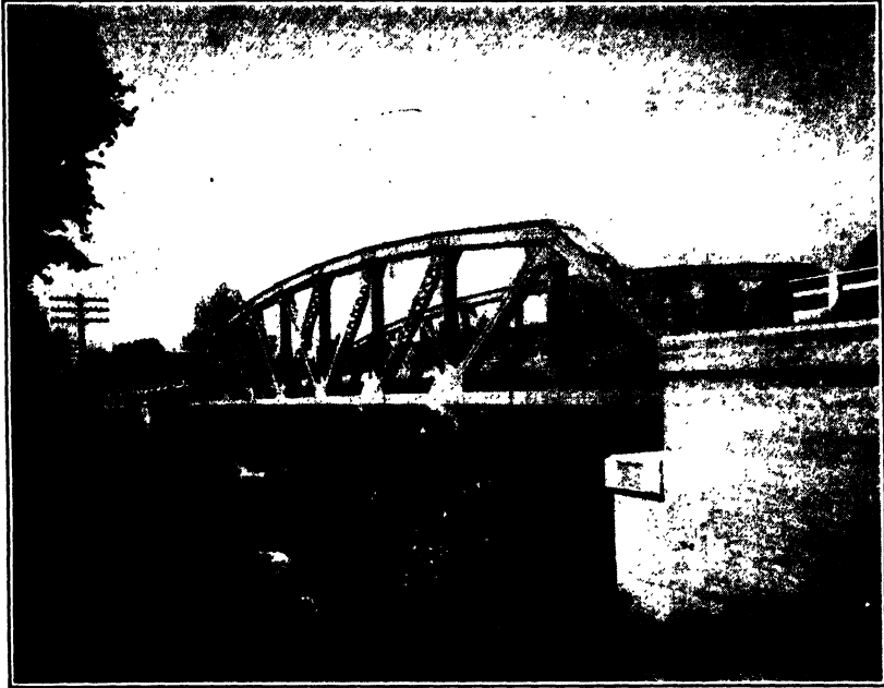
Inclined Chord Truss.
