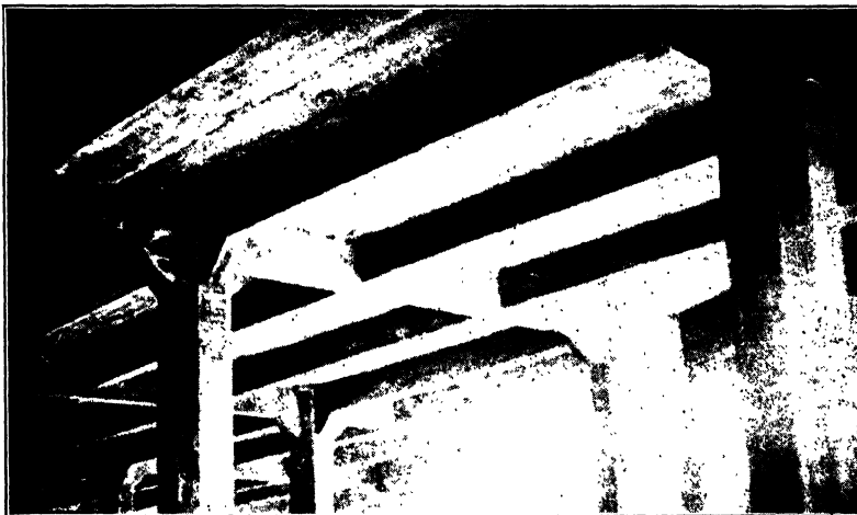
Reinforced Concrete Beam and Girder Construction.
