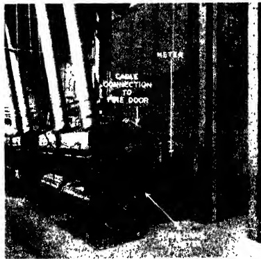
FIG. 52. LEA RECORDER ON CHAIN GRATE STOKER (Lea Recorder Co., Ltd.)
