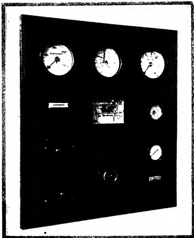
FIG. 31. MASTER PANEL FOR AUTOMATIC COMBUSTION CONTROL.
