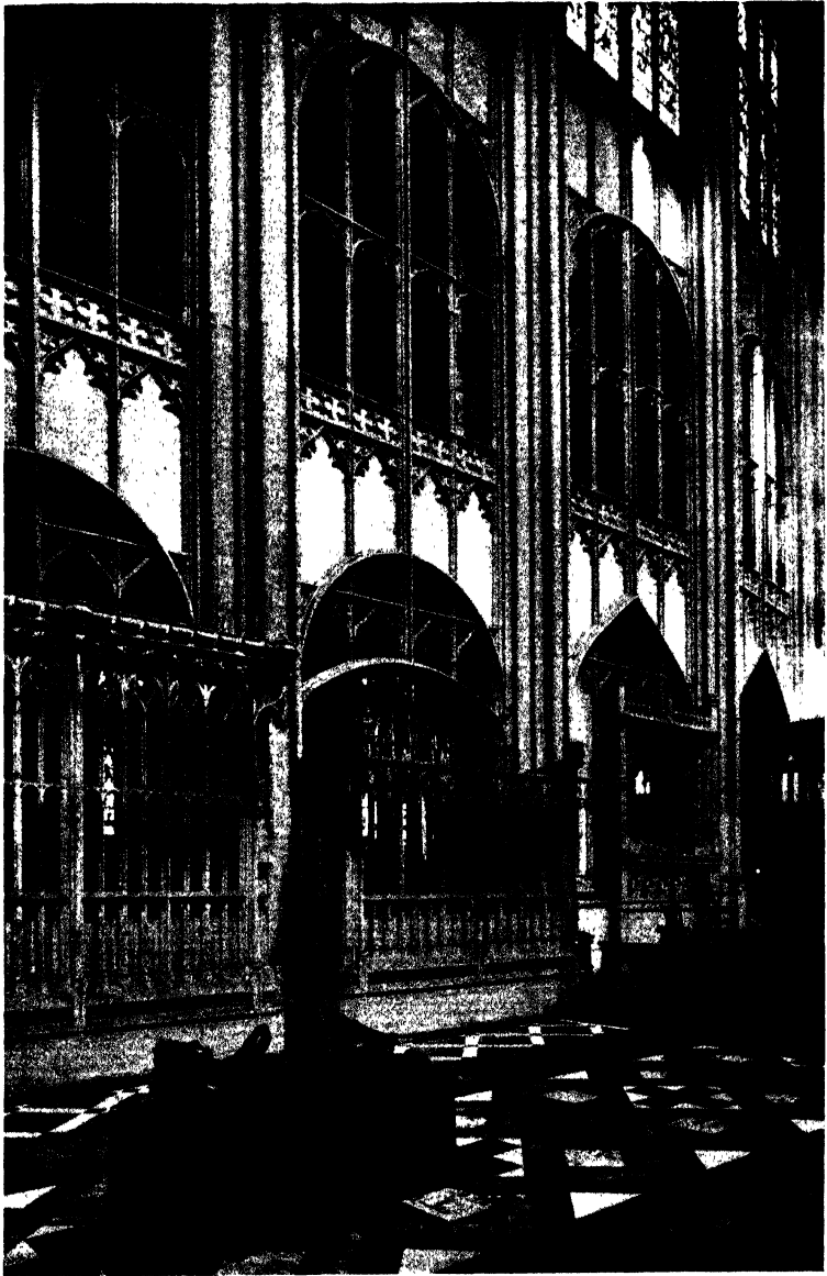
8 GLOUCESTER: A Detail of the Quire Reconstruction that worked the Perpendicular Revolution. The old Norman core is overlaid with a delicate rectilinear scaffolding of light masonry. The shrine of Edward II can be seen screened off in the central bay, and in the foreground is the early effigy of Robert of Normandy
