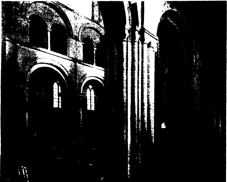
86 ROCHESTER: The Norman Arcade of the Nave
