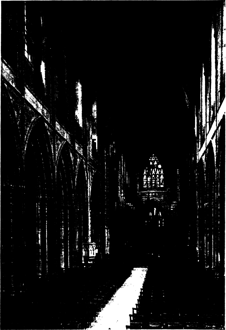
29 CHESTER: The Nave looking East, with the profile of the Return Stalls
