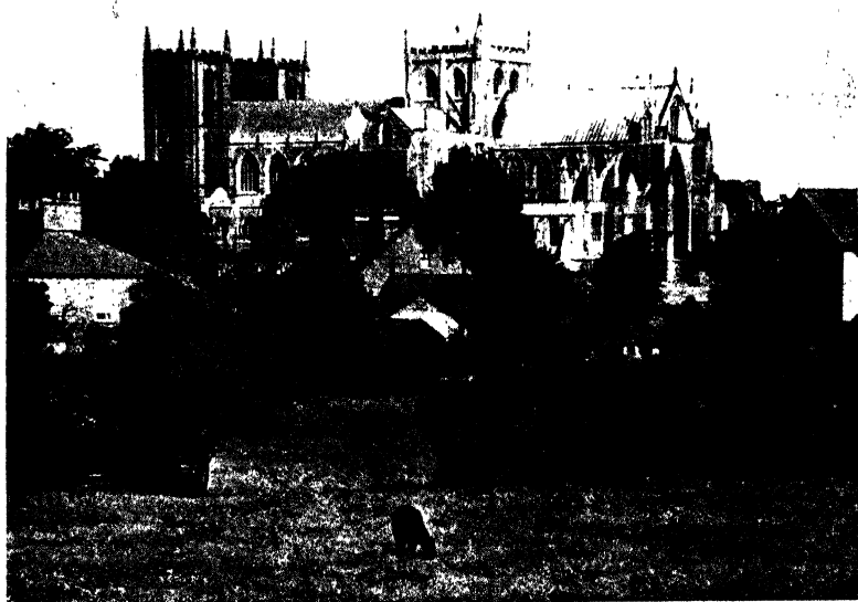
82 RIPON: The Cathedral from the South-East
