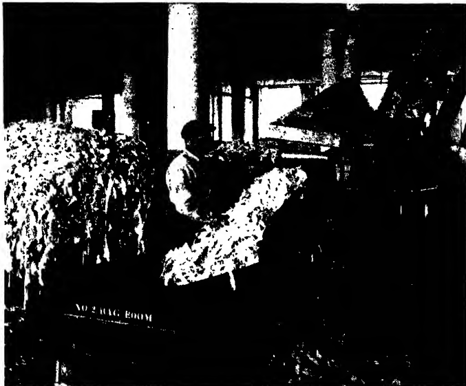
FIG. 49.—Rag cutter with conveyor feed. (Courtesy of B. F. Perkins and Son, Inc.)
