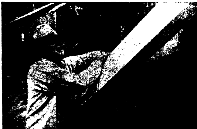
FIG. 7.—Tying on a 3- by 12-inch board. Boards and small pieces may be nailed together. (Courtesy of George O. Argall, Jr.)
