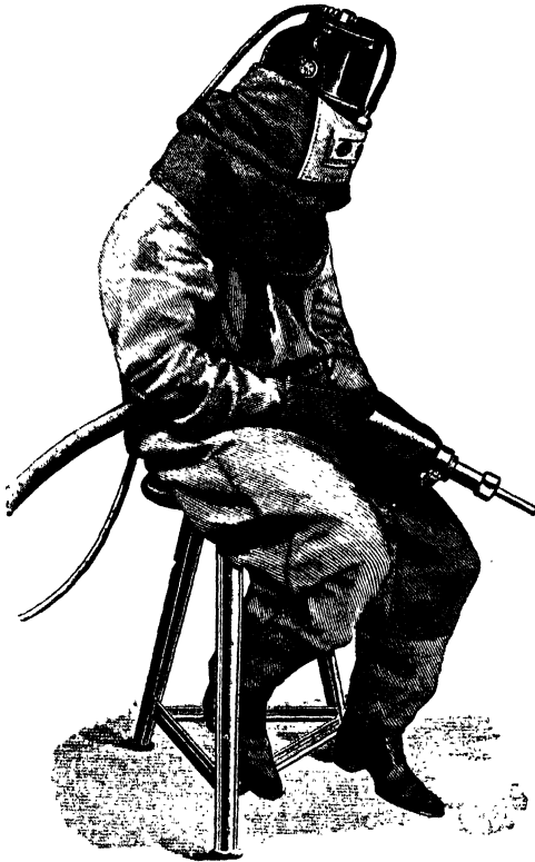
FIG. 91.—Complete Uniform for Sand Blasting Operatives.
