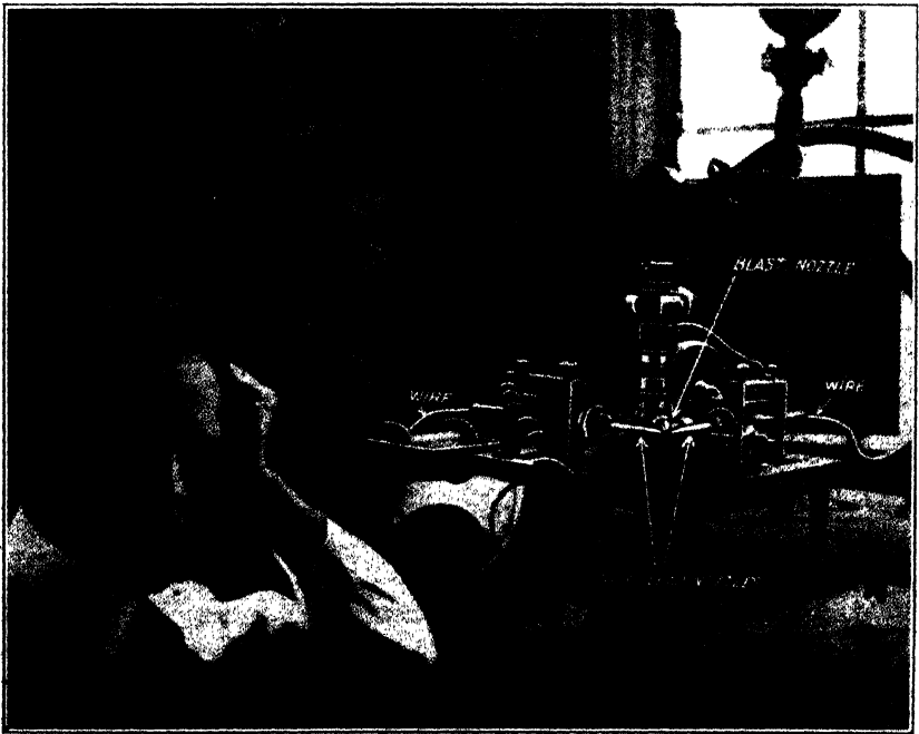
FIG. 54.—Dr. Schoop and his First Experimental Electrically-operated Metal-spraying Apparatus.
