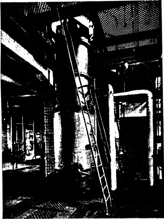
FIG. 26. Suida Plant for Acetic Acid Recovery—First Floor.
