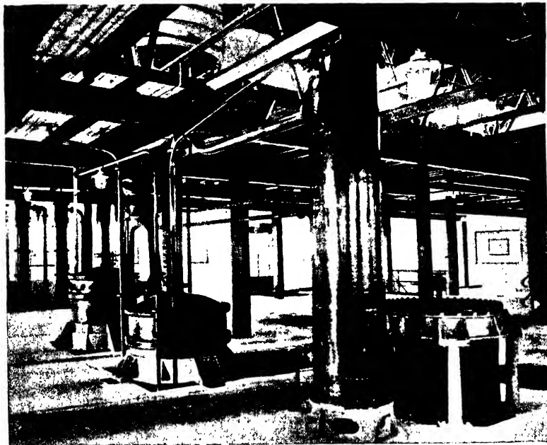
FIG. 27. Suida Plant for Acetic Acid Recovery—Top Floor.
