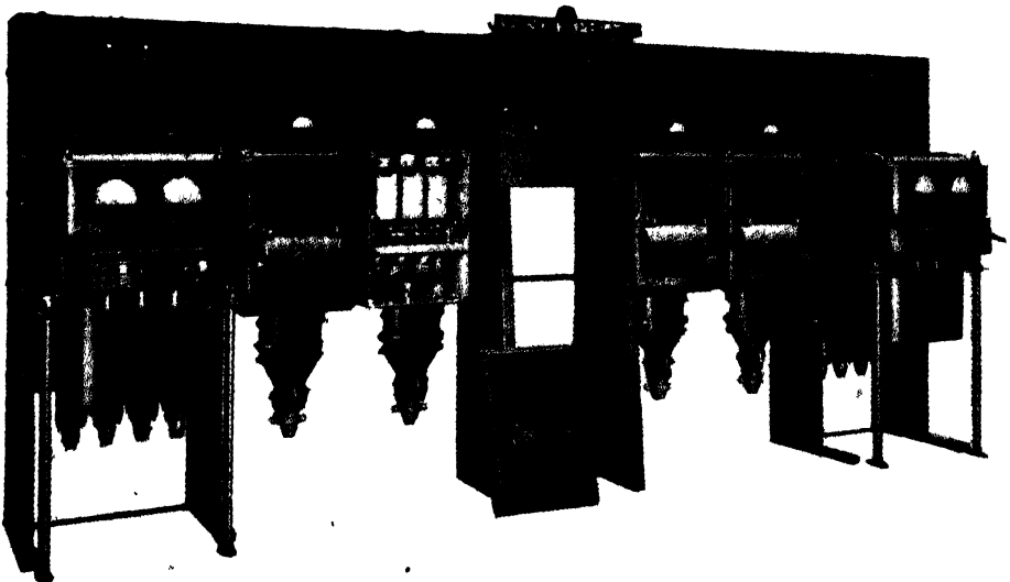
Fig. 45. —AIR-BREAK SWITCH-FUSEGEAR INCORPORATING FUSES WITH STRIKE-PIN DEVICE Two oil-immersed switches are also shown. ( Johnson & Phillips, Ltd. )
