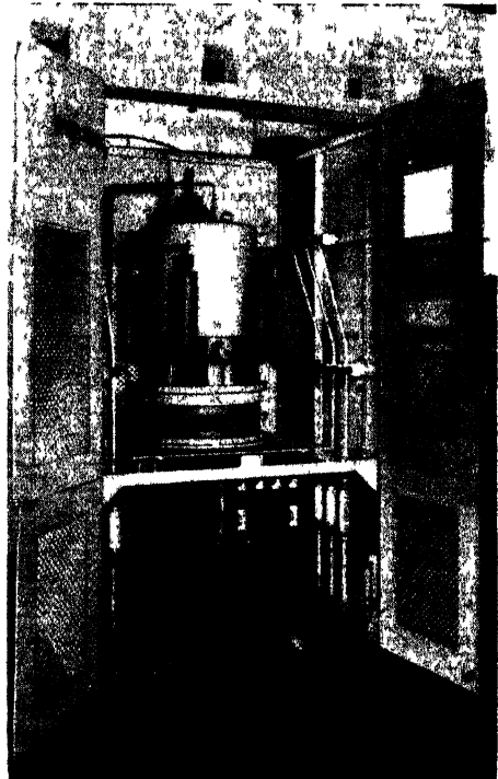
Fig. 142.—250 kW. 600 VOLTS D.C. PUMP-LESS, AIR-COOLED, STEEL-CLAD RECTIFIER EQUIPMENT (General Electric Co., Ltd.)
