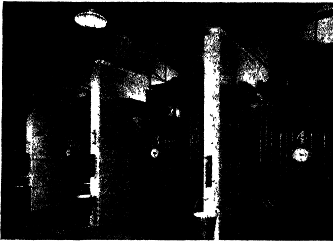
Fig. 188 —TRANSFORMERS PROTECTED BY SECTIONALISING PARTITIONS. ( Durasteel Roofs, Ltd. )
