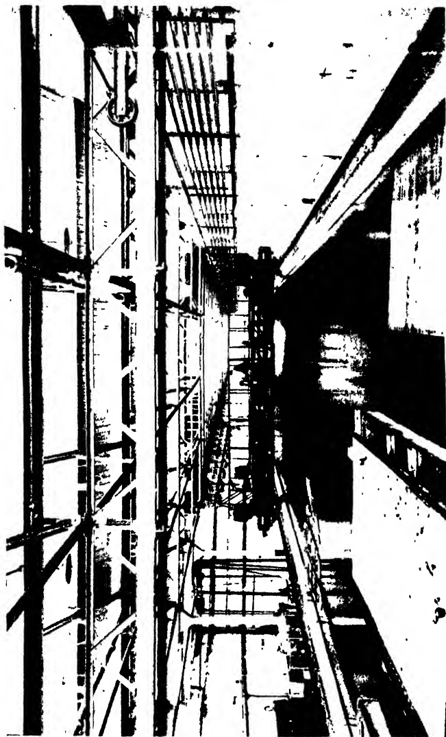
FIG. 223.— THE WILLIAM FROUDE MEMORIAL TANK : MODEL READY TO BE TOWED.
