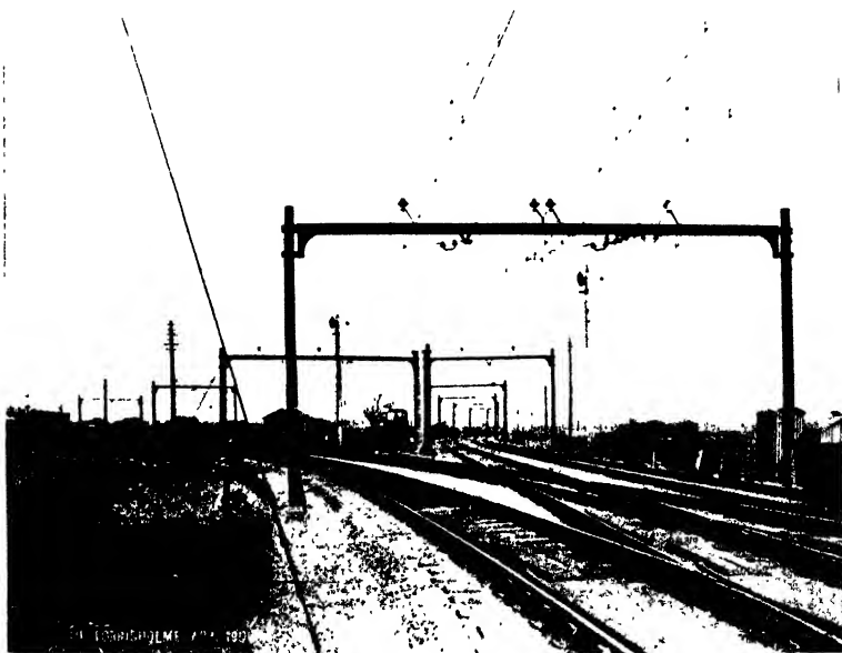
FIG. 197.—OVERHEAD EQUIPMENT AT TORRISHOLME JUNCTION (MIDLAND RAILWAY).
