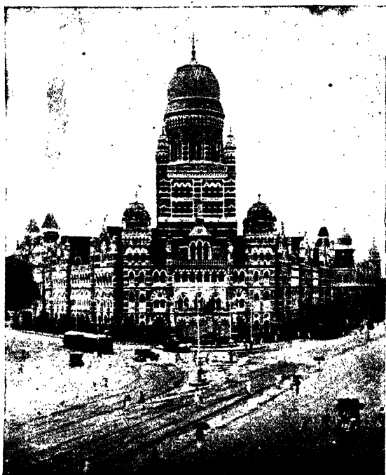
Bombay Municipal Buildings
