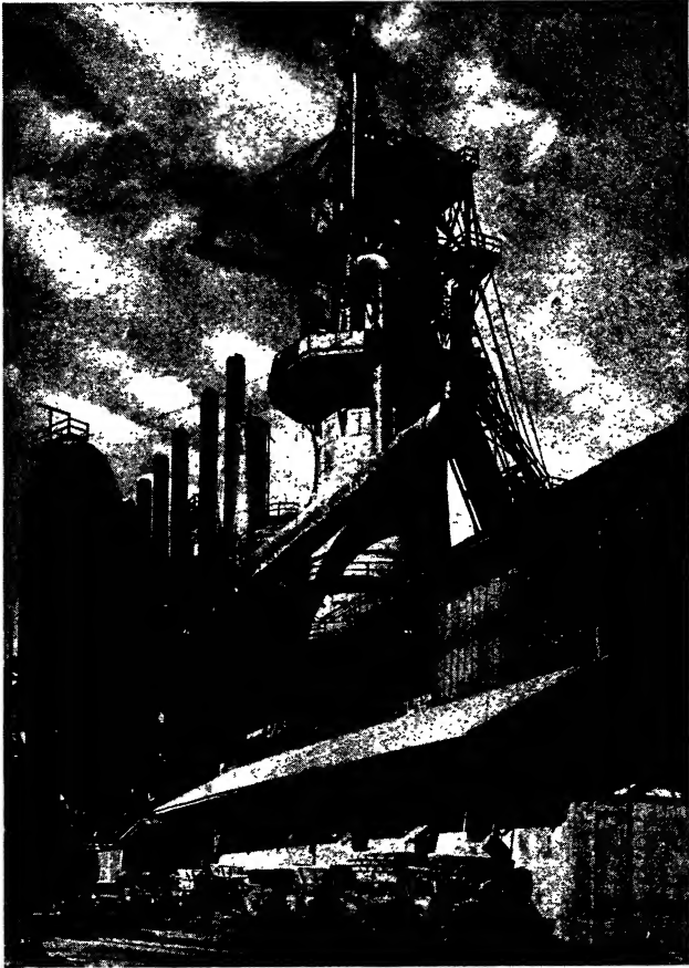
FIG. 28.—View of modern blast furnace showing elaborate superstructure. The cars containing the charge are hoisted on the inclined plane shown at the right. The gas offtakes are in the center. The dust separator is at the lower left. The stacks of the hot blast stoves are at the rear. (Courtesy Republic Steel Corporation.)
