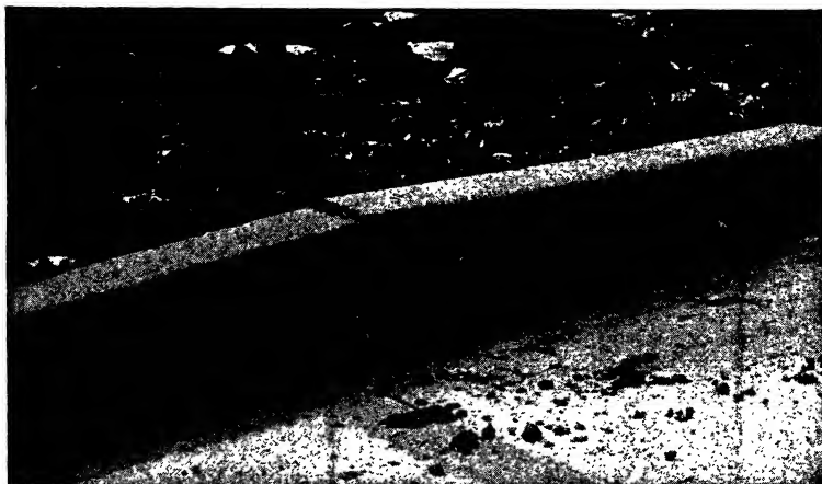
FIG. 166.—Upheaval of concrete curb due to expansion.
