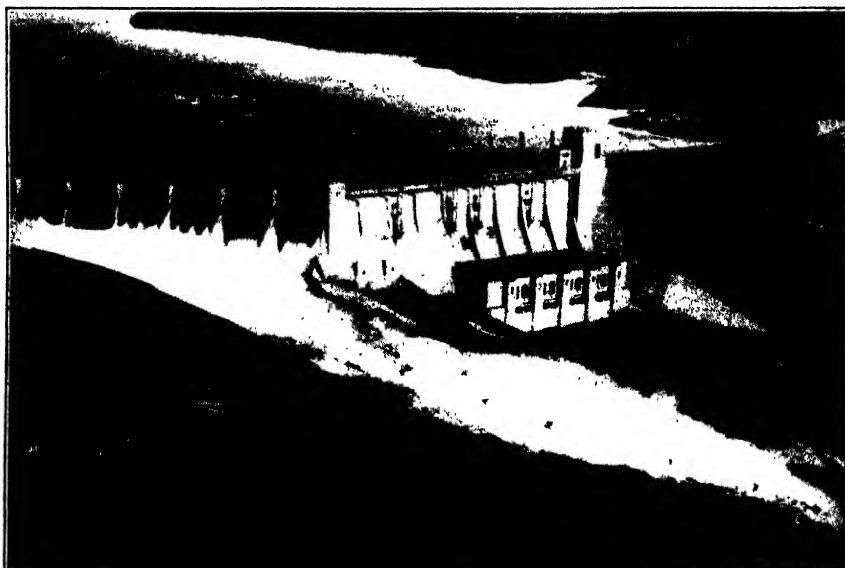
FIG. 1. Comerford Station, Monroe, New Hampshire, and Barnet, Vermont, is the largest hydroelectric plant in New England. Its four generating units have a capacity of 150,000 kilowatts. (New England Electric System, Photo by Fairchild Aerial Surveys, Inc.)
