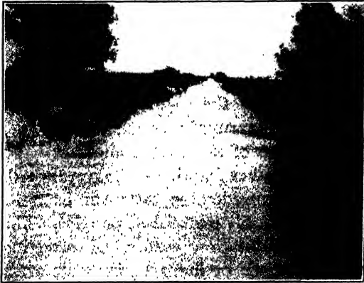
FIG. 5. The Farmers' Ditch about halfway along its 16-mile course. Like most canals, this one is an open, unlined trench.
