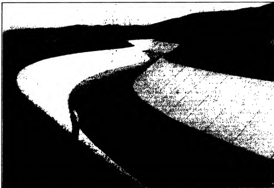
FIG. 10. Friant-Kern canal. View looking upstream along a lined section of the canal about two miles below Friant Dam. This canal is a part of the Tulare Basin District, Central Valley Project. Lined canals are necessary where permeable soils result in heavy losses of irrigation water. (Bureau of Reclamation.)
