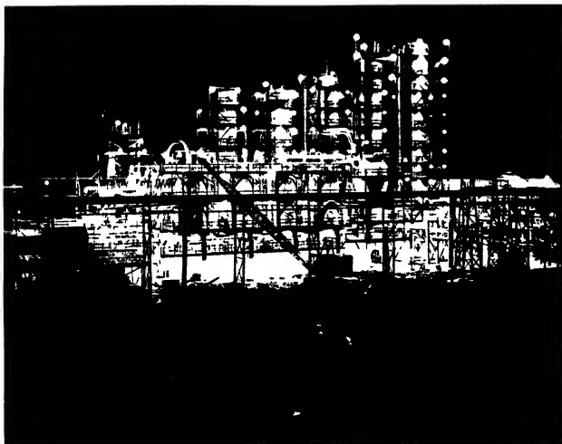
FIG. 4 Combination unit of 32,000 barrels daily capacity at Texas City, Texas, refinery of Pan-American Petroleum and Transport Company
