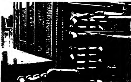
FIG. 1. Trumble heating coil from an early pipe still in a California refinery.
