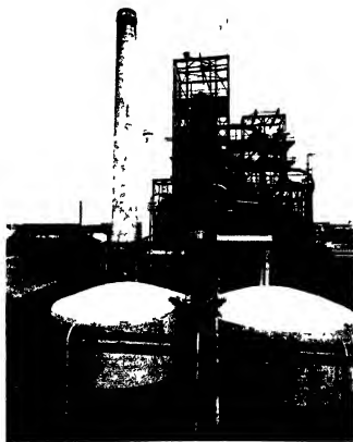
FIG. 2. A single-tower, multiple-stream pipe still of 7,500 barrels daily capacity built in 1926. In foreground, insulated tanks for hot residuum and in middle distance, with open manhole, a vacuum pot used when running crude to lubricating oil or bright stock residuum.
