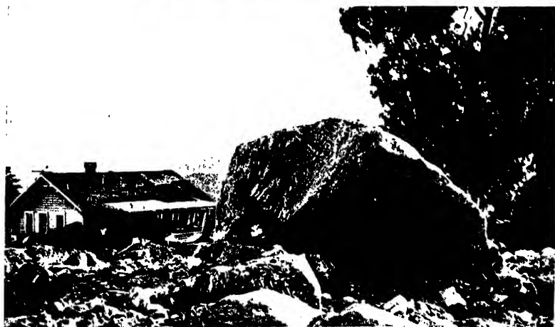
FIG. 21.—Destruction of highway-maintenance station, near La Crescenta, California, caused by flood from burned-over mountain area, Dec. 31, 1933.
