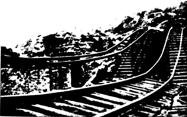
(B) Buckling of railway lines near Tokyo
