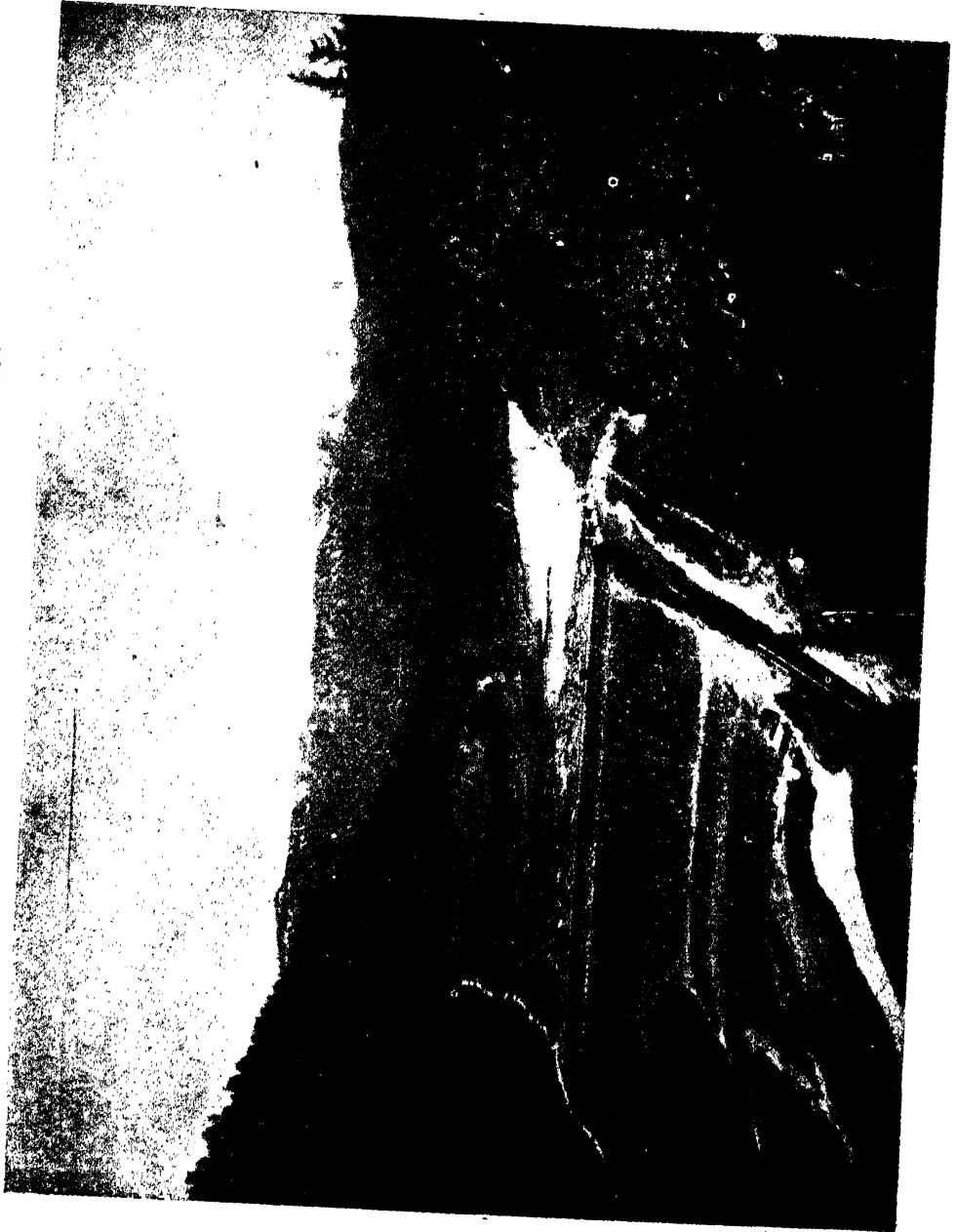
Tielon Dam, Completed in 1925, height 300 ft. Earthquake and Rock fill embankment, concrete corewall.
