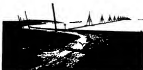
FIG. 5 Wire network lightning protection over a California oil storage reservoir
