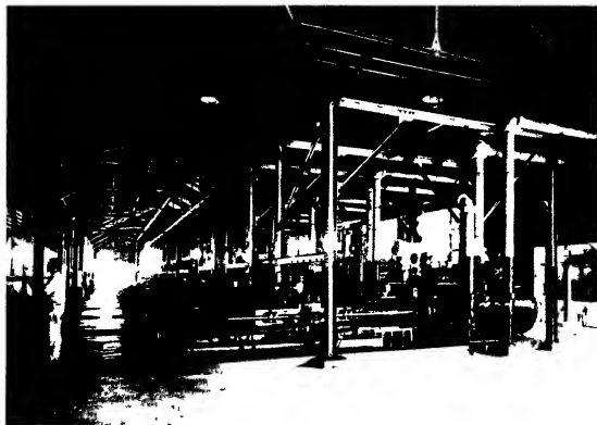
FIG. 4 High-pressure feed pumps Baton Rouge Hydrogenation Plant
