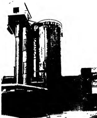
FIG. 4. Thylox liquid purification plant at Racine, Wisconsin. Left to right: thionizer, sulphur slurry tank, absorber.
