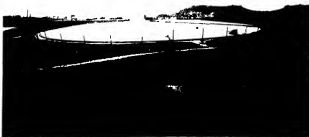
FIG. 7 Tower and wire network lightning protection over a California oil-storage reservoir
