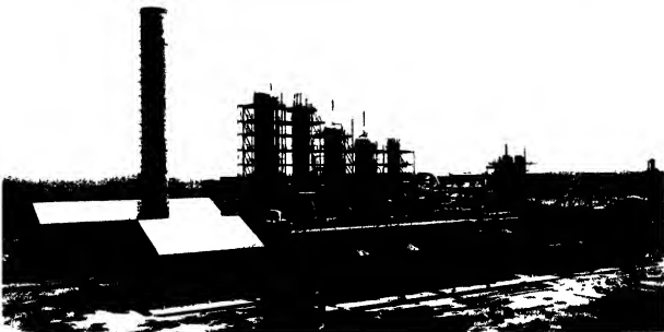
Combination cracking unit for the complete processing of crude oil to gasoline and fuel oil Throughput, 32,000 barrels per day
