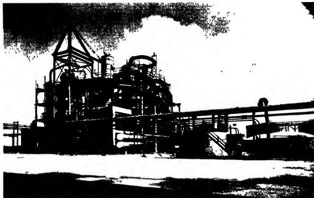
FIG. 3 Front view Duo Sol plant showing solvent recovery equipment
