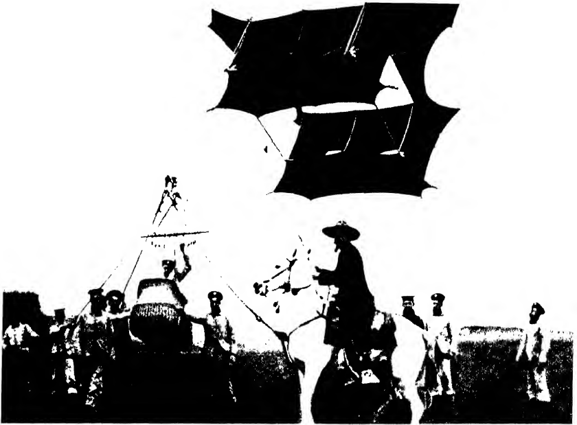
CODY MAN-LIFTING KITE, 1906. S. F. Cody interested the War Office in the possibilities of man-lifting kites of his own design. Work in connection with them was carried out under his direction at Farnborough; his picturesque mounted figure sometimes brought into the Hampshire landscape a note of the Wild West.
