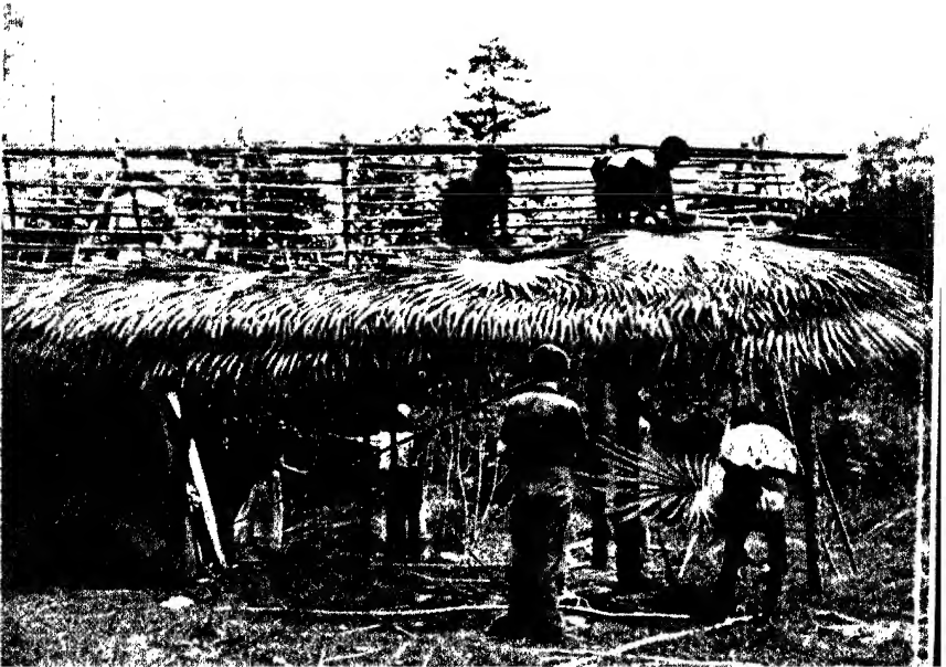
The Jicaques thatching the roof afterwards with palm leaves
