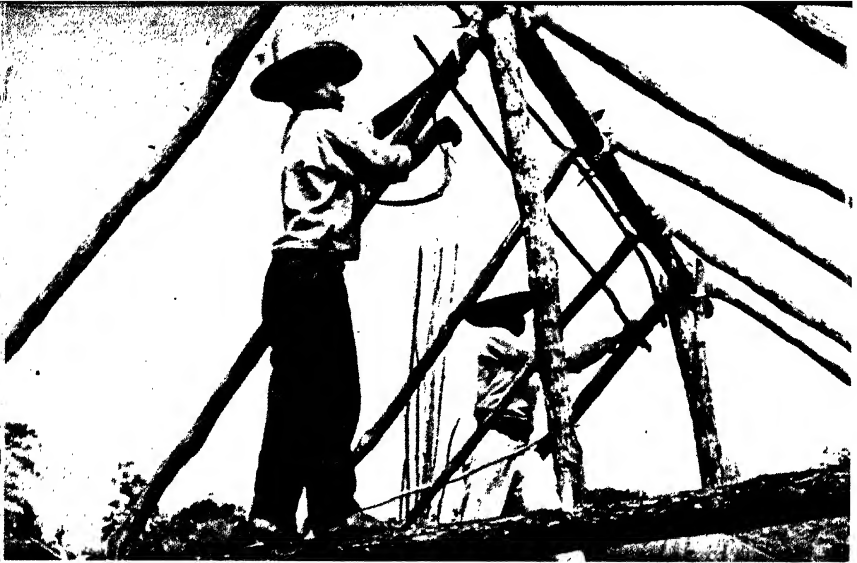
Building our house : Ramón Lopóz and his father lashing the cross-poles to the roof frame
