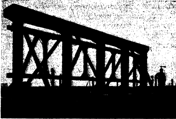
Fig. 17.—The first completely welded railway bridge of the German State Railway
