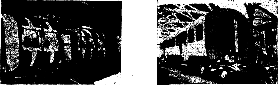
Fig. 359. Arc welding all-light-metal coaches for the Chemins de Fer du Nord.
