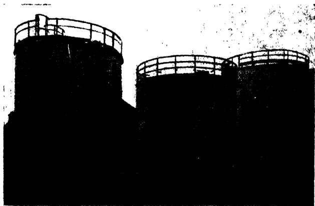
Fig. 349. Welded pure aluminium storage tanks of 70,000 to 110,000 gallons capacity (Schweisswerk Schlieven).
