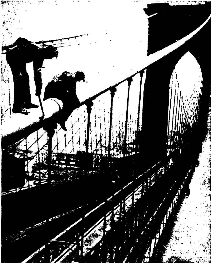
FIG. 117.—In the face of rapid strides toward laborsaving operation in most fields, painting of bridges is today practically the same operation it was 50 years ago. There has been a remarkable improvement in materials but practically none in method of applying them. This shows the maintenance painting of Brooklyn Bridge, a process which has been going ahead almost constantly during half a century.
