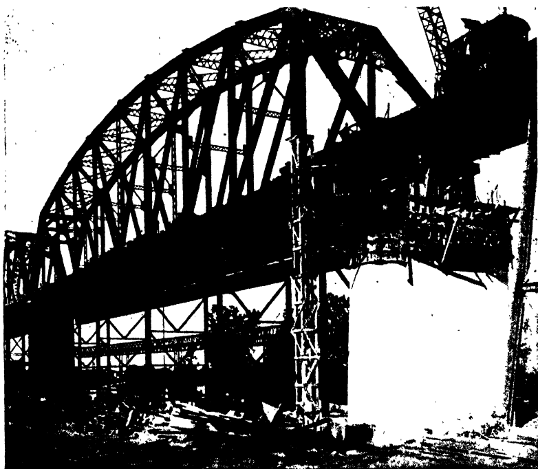
FIG. 118.—All steel bridges are carefully painted, first in the shops and then in the field. More than 10,000 lb. of red-lead paint was used for the field coats of this railroad bridge. For the field work of the George Washington Bridge more than 36,000 gal. of red-lead paint was used.
