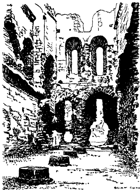
THE INTERIOR OF THE HALL, MIDDLEHAM KEEP, YORKSHIRE
