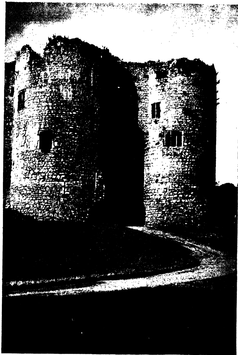
78 CHEPSTOW, MONMOUTHSHIRE: an early 13th-Century Gatehouse
