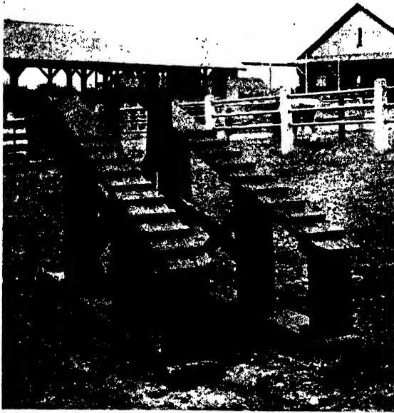
FIG. 92.—Breeding Rack. Dimensions, floor planks 9 feet long, front posts 4 feet, and rear posts 1\frac{1}{2} feet. One and one-half feet between floor planks in front and 2 feet in rear.
