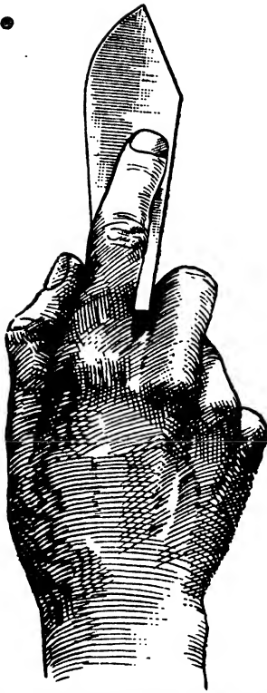
Fig. 11. Stopping must be pressed firmly into all cracks and holes, finally leveling off with the flat edge of the knife.
