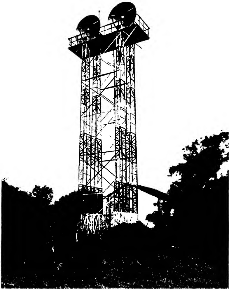
PLATE IX. PARABOLIC MIRRORS WITH HEMISPHERICAL REFLECTORS AT THE FOCUS—USED FOR CROSS-CHANNEL COMMUNICATION ON A WAVELENGTH OF 17 CM IN 1931
