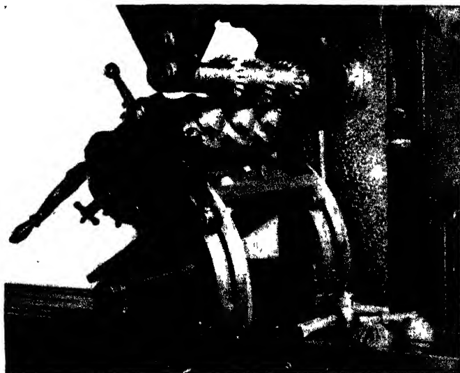
Fig. 8-14. Milling teeth in angular refacing cutters held in a specially made fixture. ( The Brown & Sharpe Manufacturing Company )
