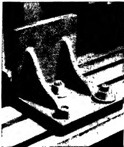
Fig. 8-24. The bolt on the left is too short and the few threads engaged in the nut can easily be stripped. (James Anderson)
