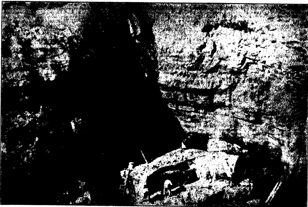
FIG. 3. PORTLAND STONE: PERRYFIELD QUARRY Showing depth of stone compared with the amount of waste or rubble
