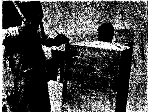
WORKING MARGINAL DRAFTS Showing method of using mallet and drafting-chisel
