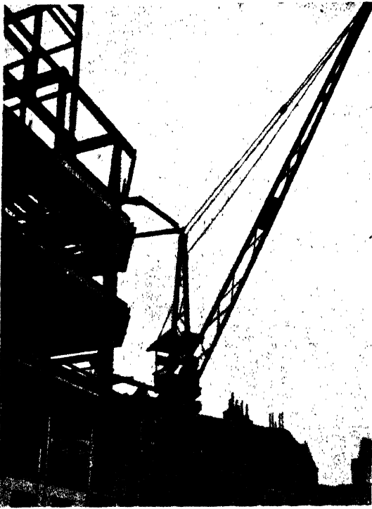
FIG. 176. CRANE FIXED TO FACE OF STEEL FRAMEWORK
