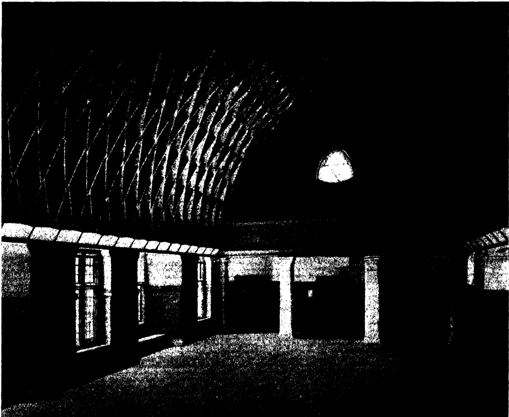
FIG. 144. CHURCH HALL ROOF
