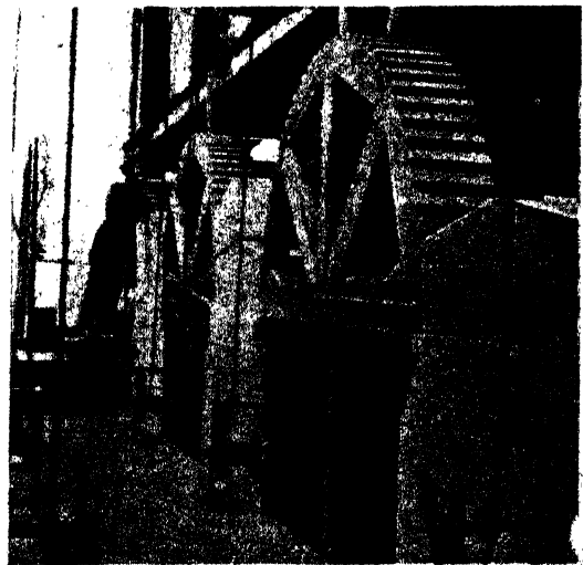
FIG. 203. CENTERING SUPPORTING MASONRY ARCHES
