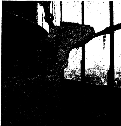
FIG. 201. ATTACHING CORNICE TO STEELWORK
