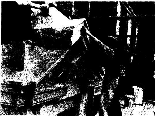
FIG. 181. PEDIMENT BEING FIXED BY MEANS OF CHAIN DOGS
