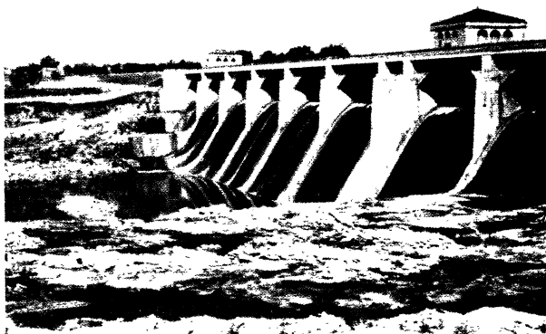
Fig. 8.—O'Shaughnessy Dam built in 1925 near Columbus, Ohio. Limestone Coarse Aggregate used. No signs of any Solution of the Stone.
