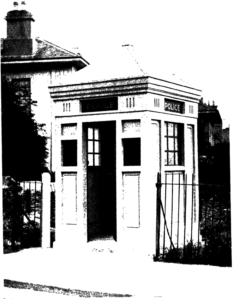
Fig. 1.—Precast Concrete Police Kiosk made with Limestone Aggregate.
