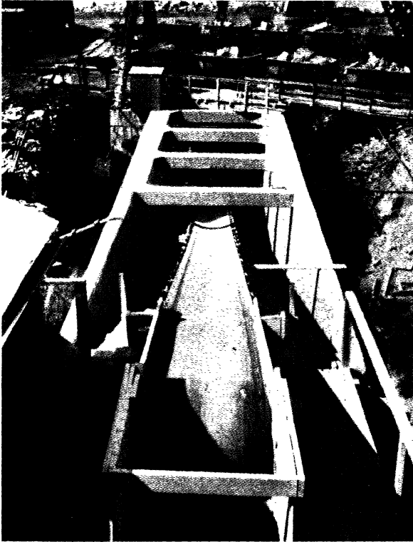
Fig. 7.—Concrete Pit, New York, built in 1924 with Limestone Fine and Coarse Aggregates. Subjected continuously to Water with no Deterioration and no Leakage.
