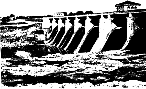
Fig. 8.—O'Shaughnessy Dam built in 1925 near Columbus, Ohio. Limestone Coarse Aggregate used. No signs of any Solution of the Stone.
