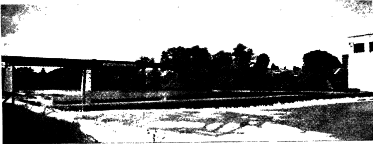
Fig. 9.—Dam at New Braunfels, Texas, built in 1922 with Limestone Coarse Aggregate. Continuously under Water with no signs of Deterioration.
