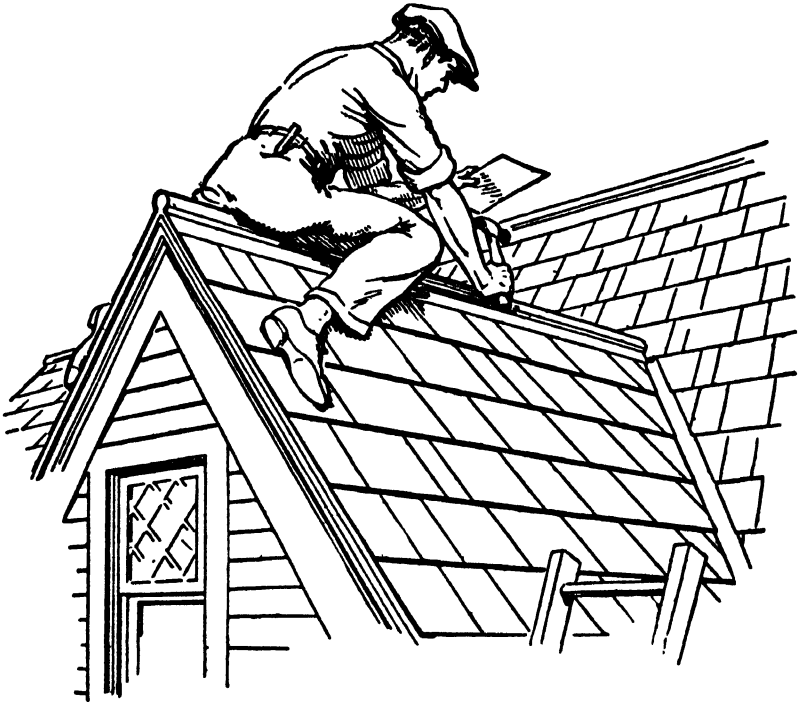
Fig. 134.—Do not attempt work of this type without sufficient protection. Use ladders, guards, roof brackets, or scaffolds where it is at all possible.
