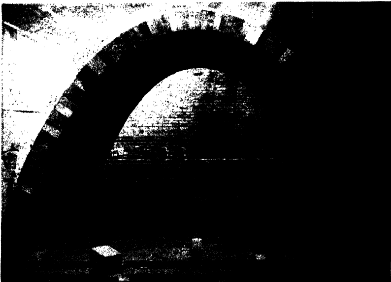
FIG. 399. Catenary. (Courtesy of Babcock & Wilcox Company.)
