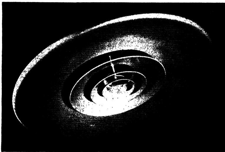
FIG. 102.—Rosette-type air-supply fitting. ( Amemostat Corporation of America. )
