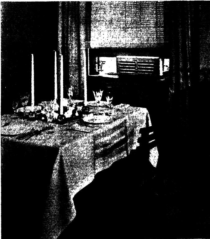
FIG. 202.—Unit ventilator with cleaner and silencer. ( American Radiator & Standard Sanitary Corporation. )
